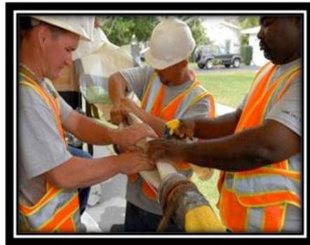
Figure 7: Inserting Liner/Bladder
