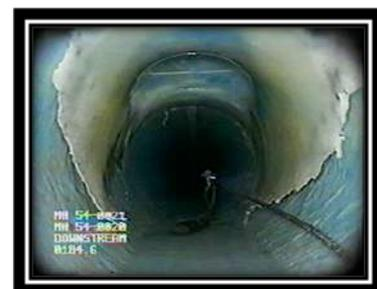
Figure 1: Delaminated
