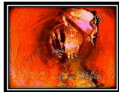
Figure 4: Protruding Hammer Tap
