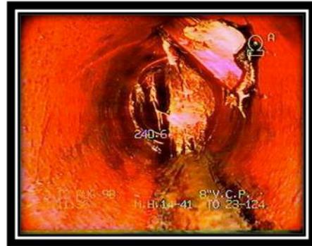
Figure 6: Protruding Hammer Tap
