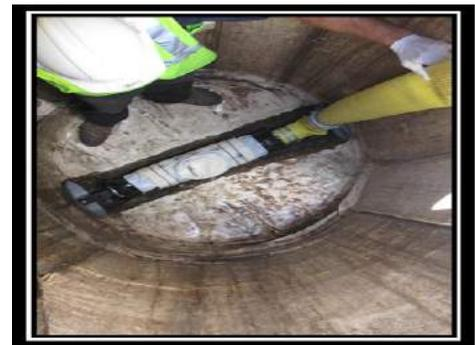
Figure 9: Inserting Launcher
